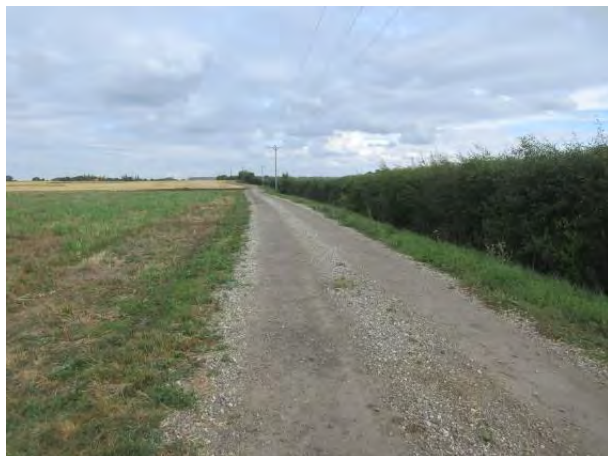
Photograph 18. Farm access track towards substation and transformer location. Load approaches camera. Negotiable with caution and confirmation of overhead clearances to power lines. Road width 3.4m.
